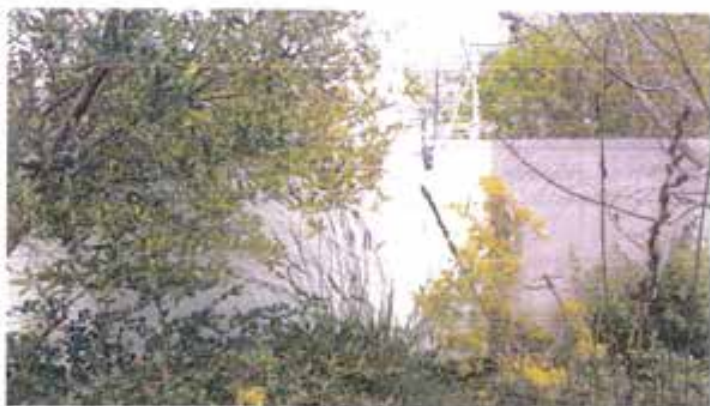
WALLS WITH ELECT. FENCE IN AREA.
