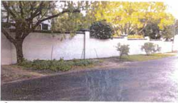
SIMILAR WALLS IN NEIGHBOURHOOD.
